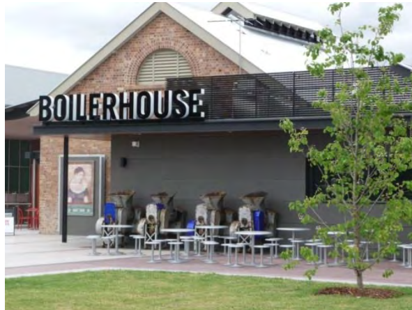
Figure 153 Former Boilerhouse at UWS Parramatta campus, Rydalmere, adaptively reused as a café, with sculptures made from former equipment. (Photo: Margaret Betteridge)
