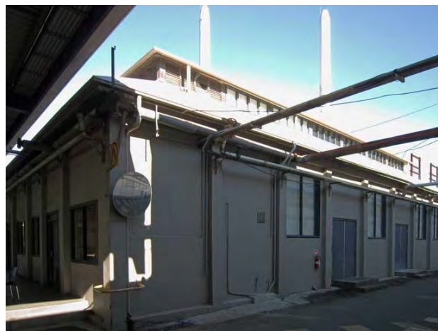
Figure 85 The exterior of the John Austin Centre, showing the early louvre panels in the clerestory. (Source: Orwell & Peter Phillips Architects)
