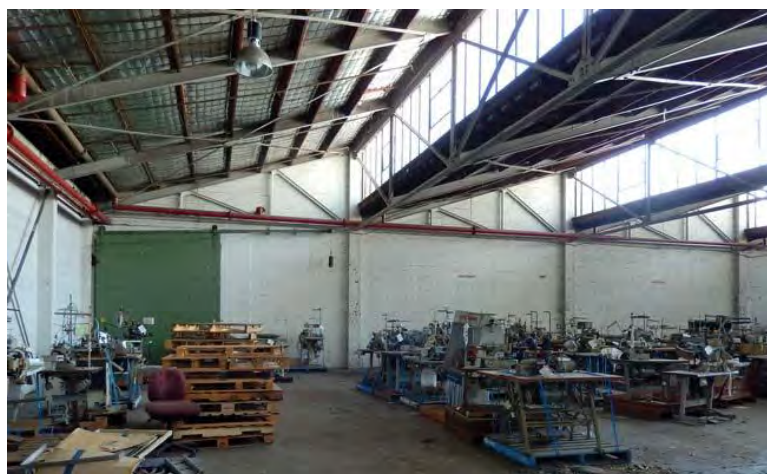
Figure 94 Interior of the New Bale Stores 2013. (Source: Orwell & Peter Phillips)
